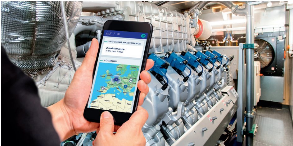
A connectivity device transmits vital equipment data in near real-time to your screen.
